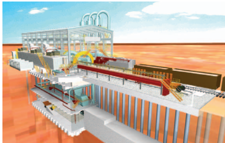
1 The car dumper was a challenging engineering exercise as the dumper was around 40 meters deep and the ground water table was around 2 meters.
